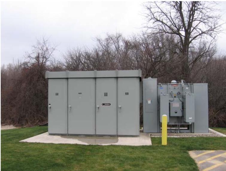
A company in Schenectady, NY needed to solve the problem of the event of a utility power outage. KJ Electric engineered the project, procured and installed the equipment, started it up and tested it. The result supplies 13.8KV to the facility in the event of a power outage.
