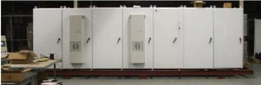
The main drive panel has 7 bays, and is NEMA 12 rated to keep copper dust out of the internal electronics. The panel has two air conditioning units to keep the equipment inside cool.
